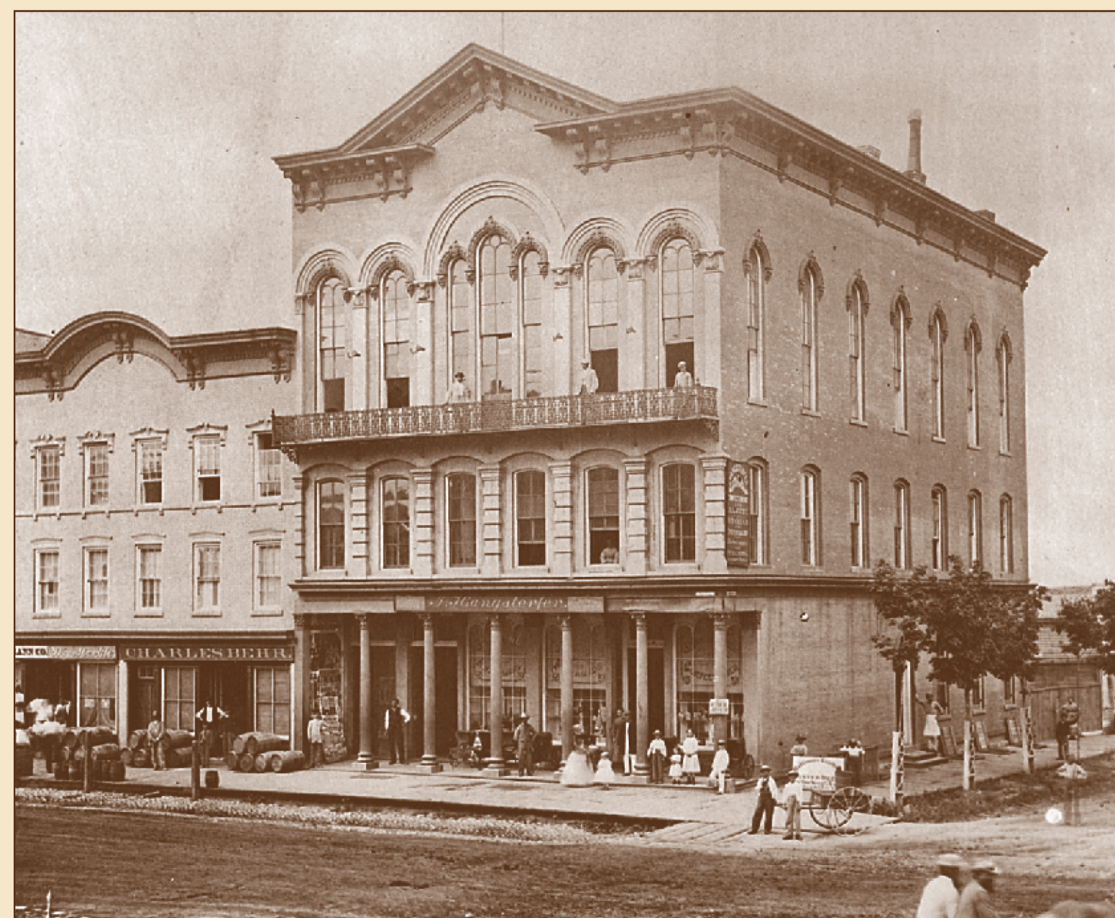
♣ Hangsterfer's Hall, on the southwest corner of Main and Washington, was torn down in 1926 for a new Kresge Dollar Store building. Mongolian Barbecue is there today.
