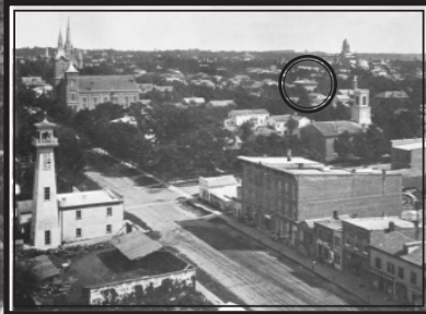
LOOKING SOUTHEAST TOWARDS CAMPUS IN 1880. BEYOND THE WATTS HOUSE (CIRCLED) IS THE DOME OF UNIVERSITY HALL ON THE HORIZON. NOTE THE NEIGHBORHOOD'S MANY CHURCH STEEPLES. THE OLD WOODEN FIRE-MEN'S HALL AT FIFTH AND HURON IS AT LEFT.
