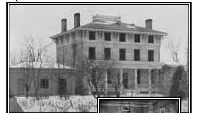
PRESIDENT'S HOUSE FROM CAMPUS, 1870s ONE OF THE FOUR FACULTY HOUSES BUILT IN 1840 BECAME THE PRESIDENT'S HOUSE WHEN HENRY P. TAPPAN ARRIVED IN 1852. IT IS THE ONLY SURVIVING ORIGINAL CAMPUS BUILDING. THE THIRD FLOOR AND KITCHEN WING WERE ADDED BEFORE 1871, WHEN JAMES B. ANGELL MADE INDOOR PLUMBING A REQUIREMENT FOR ACCEPTING THE PRESIDENCY. THE CAMPUS SIDE INCLUDED BARN, AN ORCHARD, AND A VEGETABLE GARDEN.
