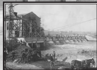
BARTON DAM UNDER CONSTRUCTION, 1912
