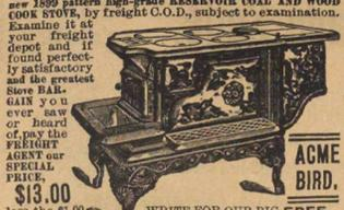
WRITE FOR OUR BIG FREE STOVE CATALOGUE. This stove is size No. 2, oven is 40x36x14, top is 42x22, made from best pig iron, extra large flues, heavy covers, heavy linings and grates.
