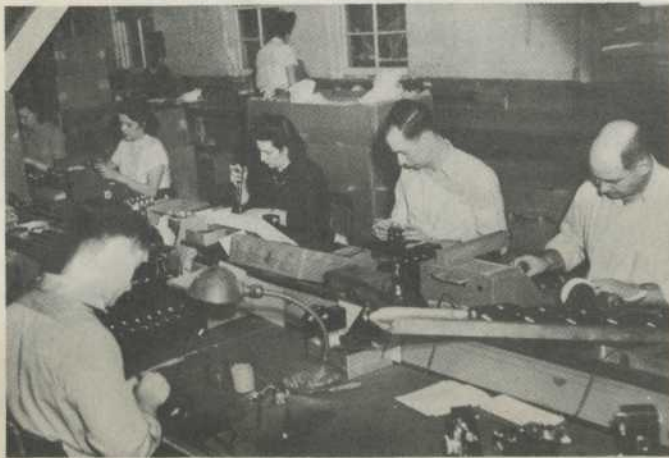
A VIEW OF THE C-3 LINE WHERE THE SHUTTER IS BEING ASSEMBLED AND ADJUSTED.
