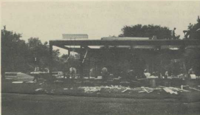
Steel framework for second floor.
