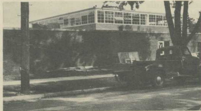
Windows complete inclosure.
