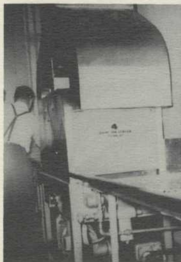
Erv Braatz supervises the installing of the automatic dishwasher.
