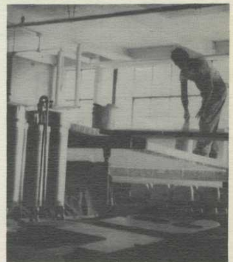
The ceiling is painted.
