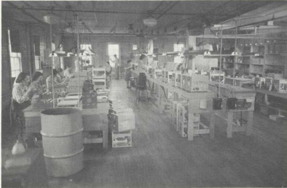
This picture, taken in the late thirties, shows one of the radio assembly lines in Plant I.
